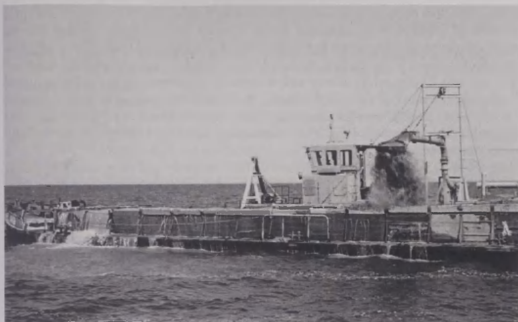
Fig. 3. Excavation of sand near Piirissaar Island. Photo by A. Raukas.
