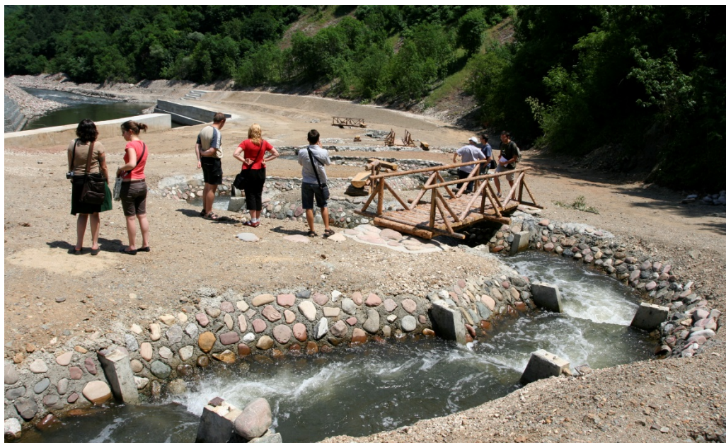
Field trip to Sovage hydro power plant, surveying fish ladder (01.07.2008).
