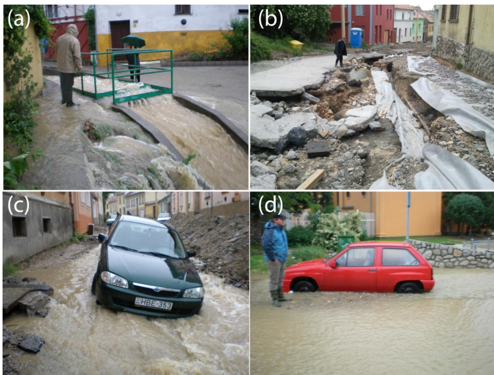
Figure 3. Damage and losses in the Vince Street on May 17, 2010. (a) the clogged drainage filter at the northern end of the street; (b) and (c): the damaged road surfaces; (d) the accumulation of deposits at the southern end of the street and the Ágoston Square
