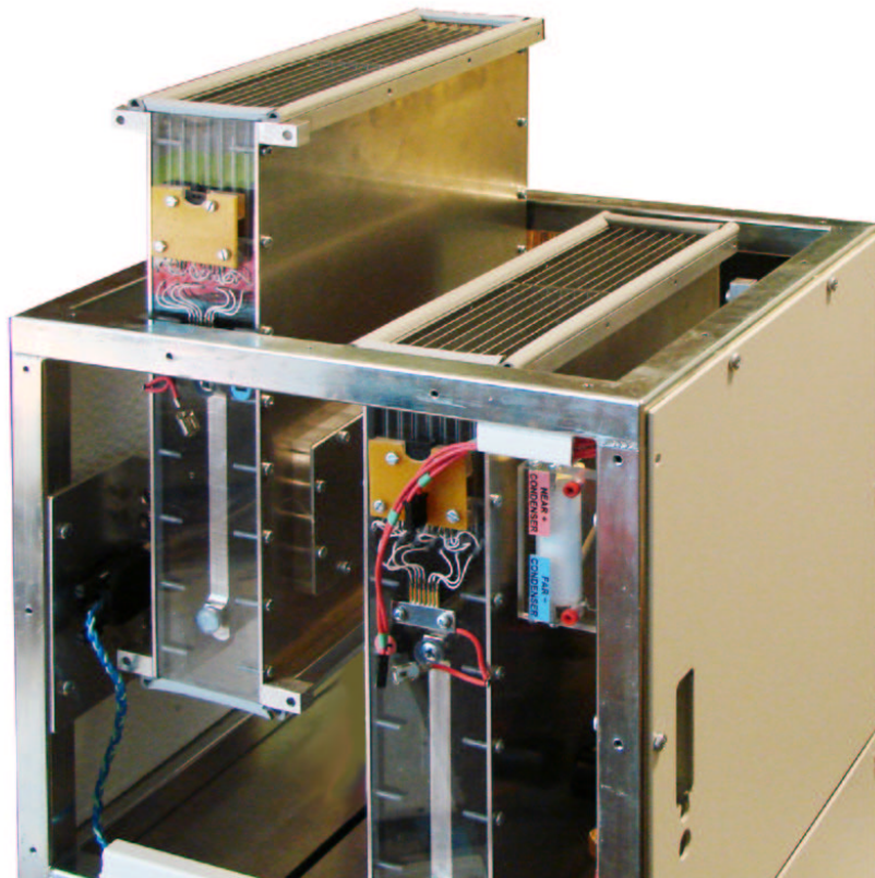
Figure. 8.5. Removing of an aspiration condenser from BSMA3.
