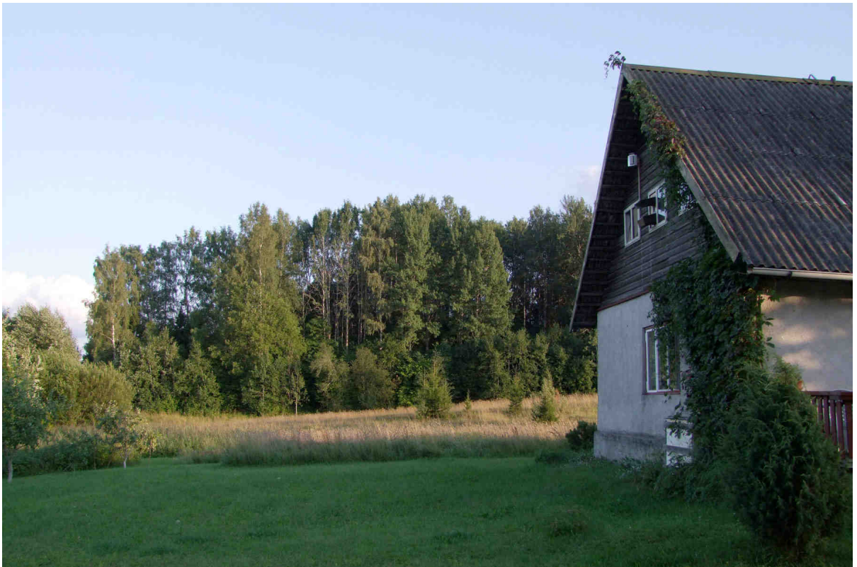
Figure A6.2. Cottage Tammemäe and the SIGMA air inlet in the center of the gable.
