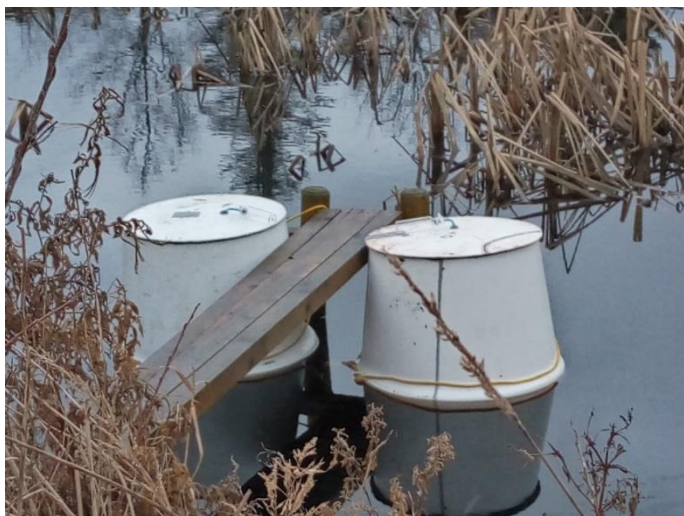
Figure 4: Installed chambers on site.
