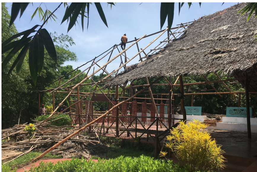
Fig. 11. The process of building a large canopy, Zanzibar (Photo: I. Khrustaleva).
