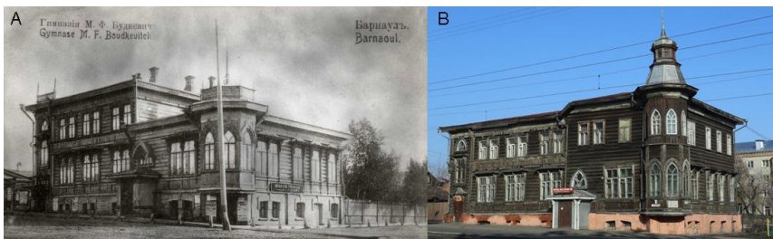
Fig. 13. Maria F. Budkevich Women's Gymnasium, an architectural monument of the early 20 th century in Barnaul, Altai Krai, Russia. A – View of the building at the beginning of the 20 th century on a postcard (image source: Altapress.ru); B – View of the building in 2021: the increase in the cultural layer is between 0.5 and 1 m and the entrance and windows of the ground floor are now covered with earth (image source: Runews24.ru).
