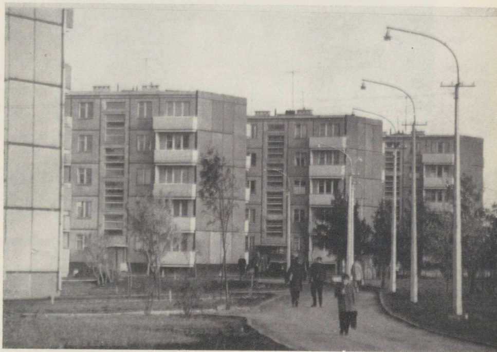
Prefabricated apartment houses at Tallinn-Mustamäe.
