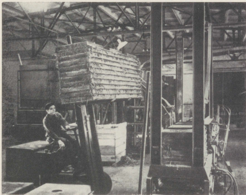
Mechanized production of TEP warmth-insulation panels.
