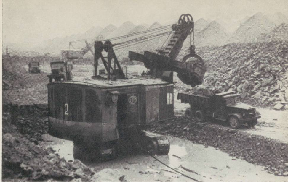
Excavator at work in the oil-shale basin.
