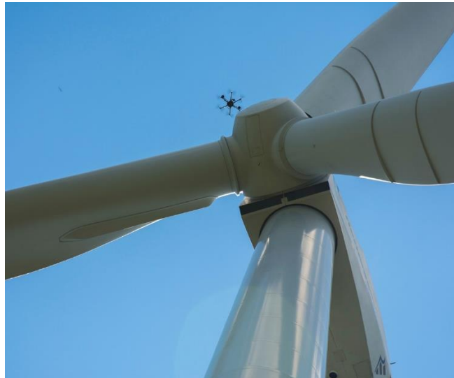
Figure 7. Inspection using an UAV [17]
