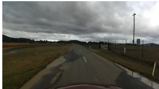
(b) On-road water hazard
