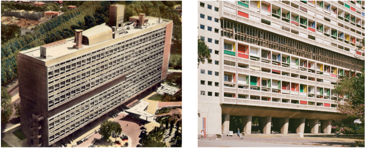
Figure.1 Unité d'Habitation in Marseille (Completed in 1952)
