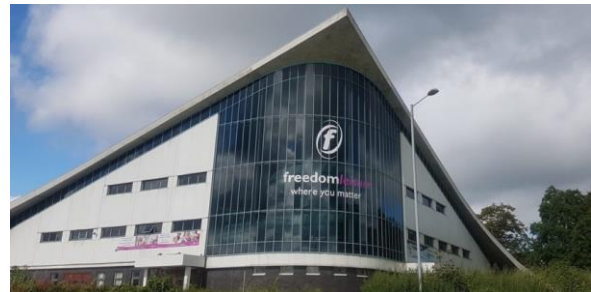
Wrexham Waterworld (Wrexham.com 2019), believed to possess the only hyperbolic paraboloid roof in Wales (Twentieth Century Society 2022).
