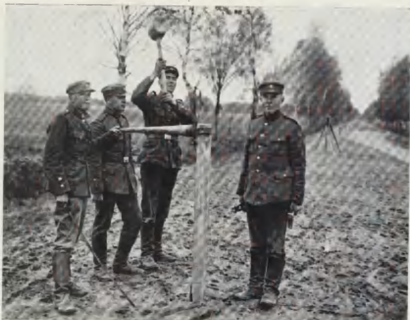
Setting of pole.
