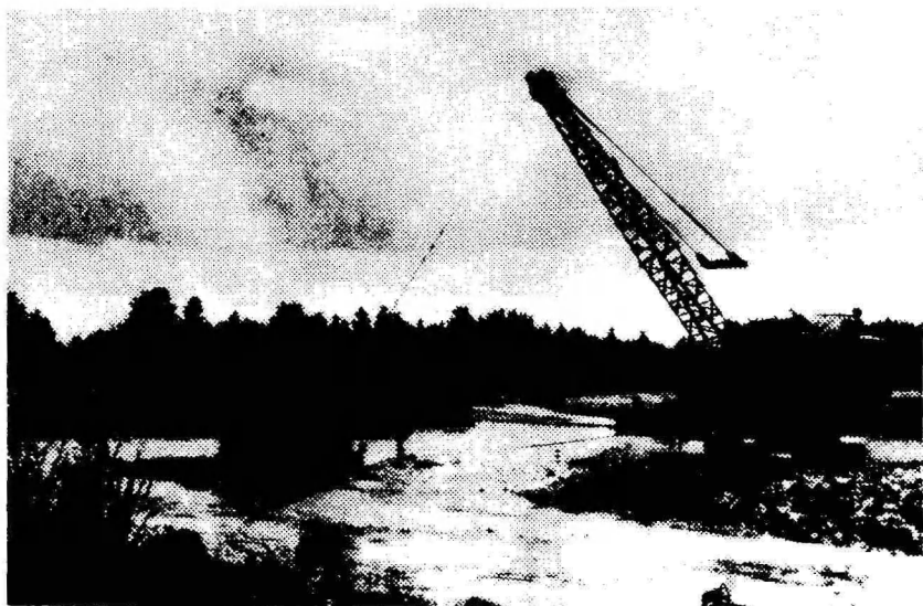
Photo 6. Land improvement: dredging of the Loobu River, North Estonia. Photo by I. Kala.
