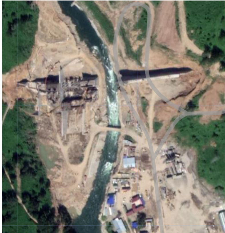
The Turgusen-1 dam as seen from remote sensing data taken from Google Earth Engine (Source: JRC imagery. Data retrieved from European Commission, processed via Google Earth Engine. Coordinates 53°09'48"N 63°36'59"E)
