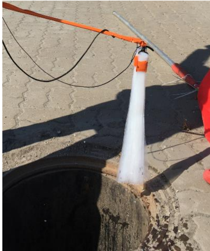
Photo 3. Biofilm carriers made of polyethylene strips were placed in the sewer
